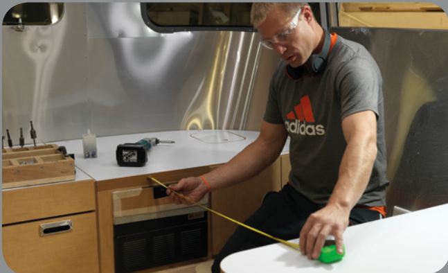
Each piece of handcrafted furniture is finished and installed by expert technicians
